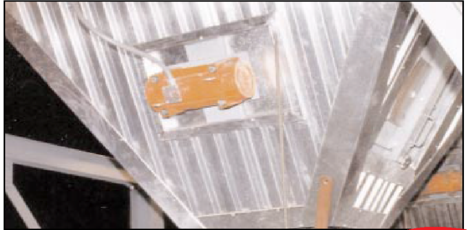
• SCR-500 on heat mount on hot ash bins
